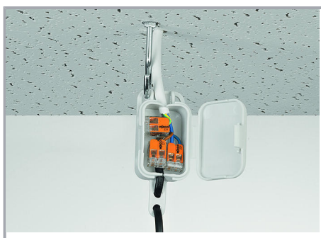
Pendant light connection in suspended ceilings
